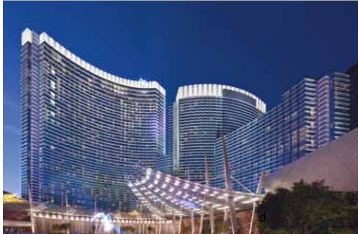
The illuminated crown elements wrap around the top 36' of each 600' tall tower, creating a signature presence on the Las Vegas skyline.
