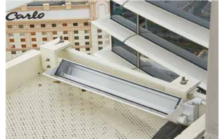
To meet OSHA fall arrest requirements and for relamping with tool-less entry, each F164 is equipped with a snap-on lens compression fitted over the extruded fixture body and tethered to the fixture by a small stainless steel cable.
