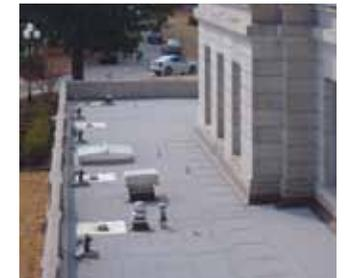
Surface mounted **M454s** with external "feet" were used at building setbacks. Units on slipfitters (not shown) were used at limited lawn mounting locations.
