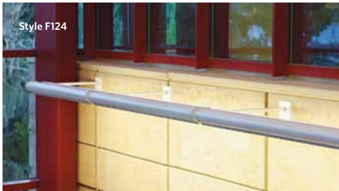
Cantilevered F124 wall washers for the side feature walls are through-wired, requiring only a single electrical feed for each row.
