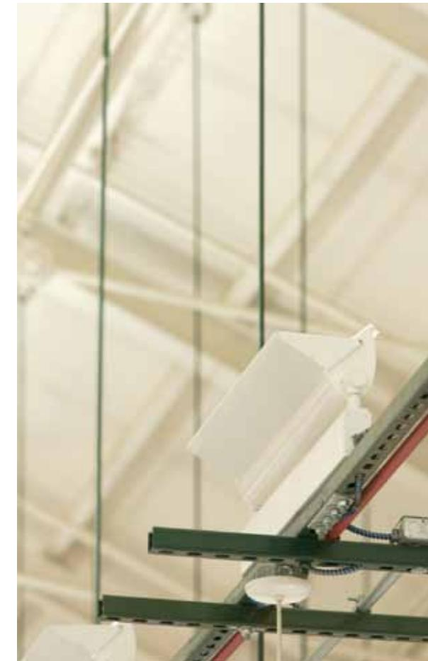
A combination of 2 ft. and 8 ft. fixtures were used to coordinate with structural spacings. The modified mounting channel on the **Style F124** mates with the Unistrut and accepts the conduit feed through an access cover on the back.
