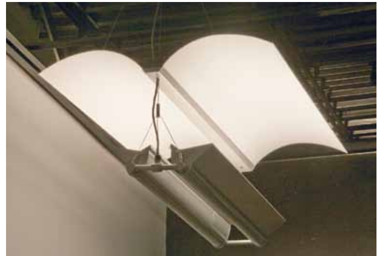
A matte powder paint finish on the custom gullwings enhances the perception of a soft, uniform glow.
