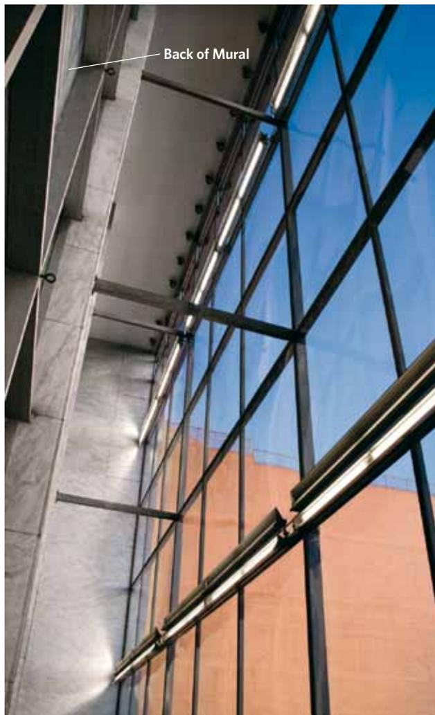
Both horizontal fixture runs utilize back-to-back reflectors, cross-firing light up and down the backside of the mural. The selected mounting locations help minimize potential shadowing from the art's structural support framing. Cutoff visors provide additional shielding for visitors who pass beneath the art.
