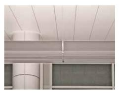
The modified **F139s** are modular in length (96") with discrete support details at joints.
