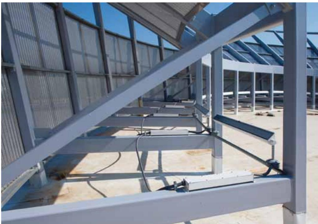
**F151s** are surface mounted to the structural frame using contractor-provided junction boxes and conduit. Remote ballast boxes are powder coated to match the fixtures.
