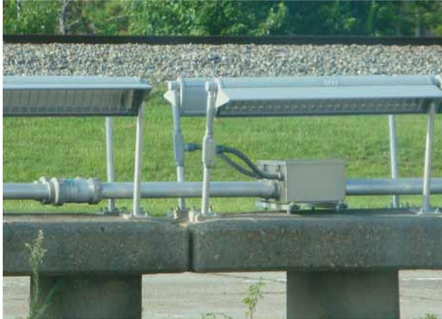
The **Style F164** reflector and visor are made of extruded aluminum. All other components are non-corrosive stainless steel or aluminum. The polyester powder coat finish exceeds ASTM's B117-90 1000 hour salt spray test. The snap-on, UV stabilized acrylic lens is impact resistant. The fixtures are sealed with silicone gasketing. Aluminum mounting hubs were supplied by The Lighting Quotient; rigid conduit support bases were provided by others.
