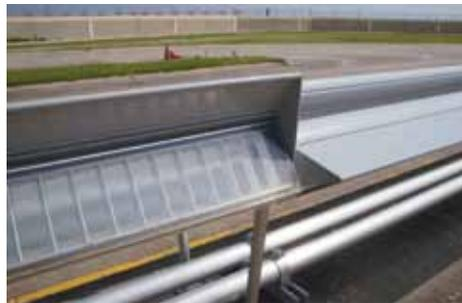
Use of an internal cross-baffle (visible in left-hand fixture, prior to final aiming) enhances lateral shielding.
