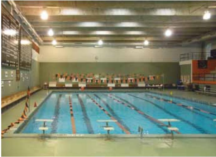
**Before:** Direct prismatic high-bays located around the edges of the pool subjected swimmers and spectators to direct glare.
