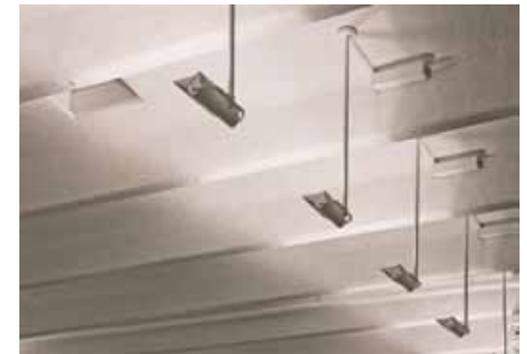
Remote ballast boxes minimize the scale of the suspended uplights, which are painted with the same powdercoat finish.
