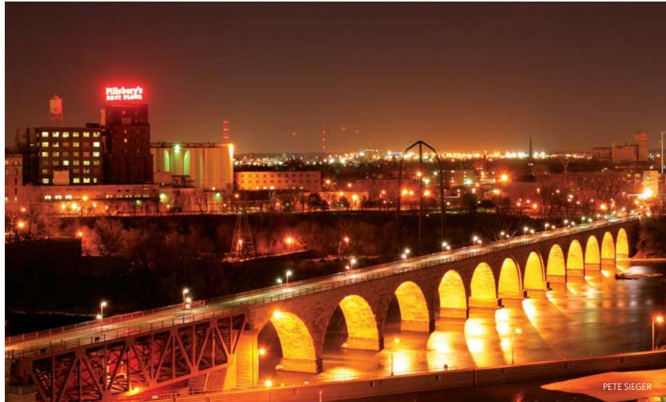
A graceful curved visage by day, until recently the bridge's arches virtually disappeared by night. The decision to illuminate the granite and limestone surfaces presented the lighting designer with several challenges. There was to be no drilling into the stone and no exposed conduit. Also, luminaires could not be located at the bases of the arches because of the potential for flooding.
