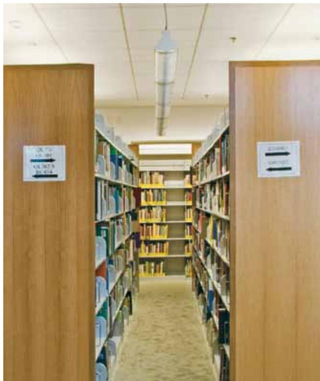
The **Style 3030** is designed to be surface, cable or stem mounted. Optional through wiring with quick connects and integral emergency battery packs were specified for TRCC.
