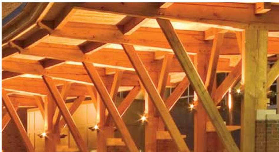
3000K pulse start ceramic metal halide lamps enhance the warm character of the wood canopy. The use of long-distance remote ballasts helps minimize the presence of the back-to-back uplights.
